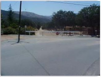
Blocking public access. KC Zoning Code Violation § 19.02.060
